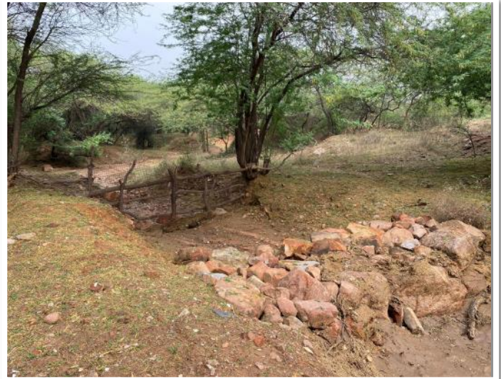
Gully plugs constructed in existing waterbodies
